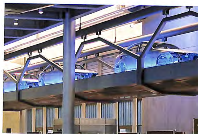
BMW plant Leipzig – central building
